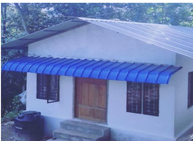
New Church Building at Manimala
