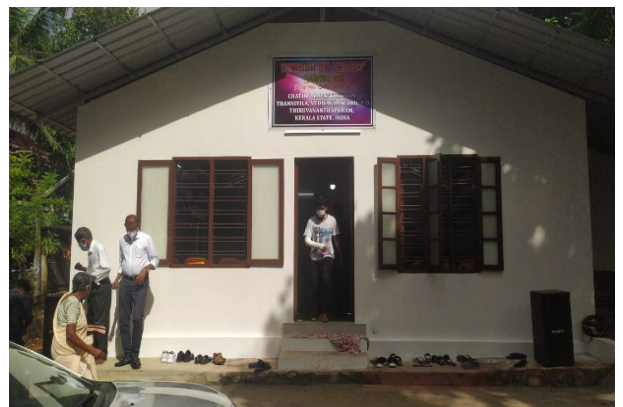
New Church Building at Trivandrum
